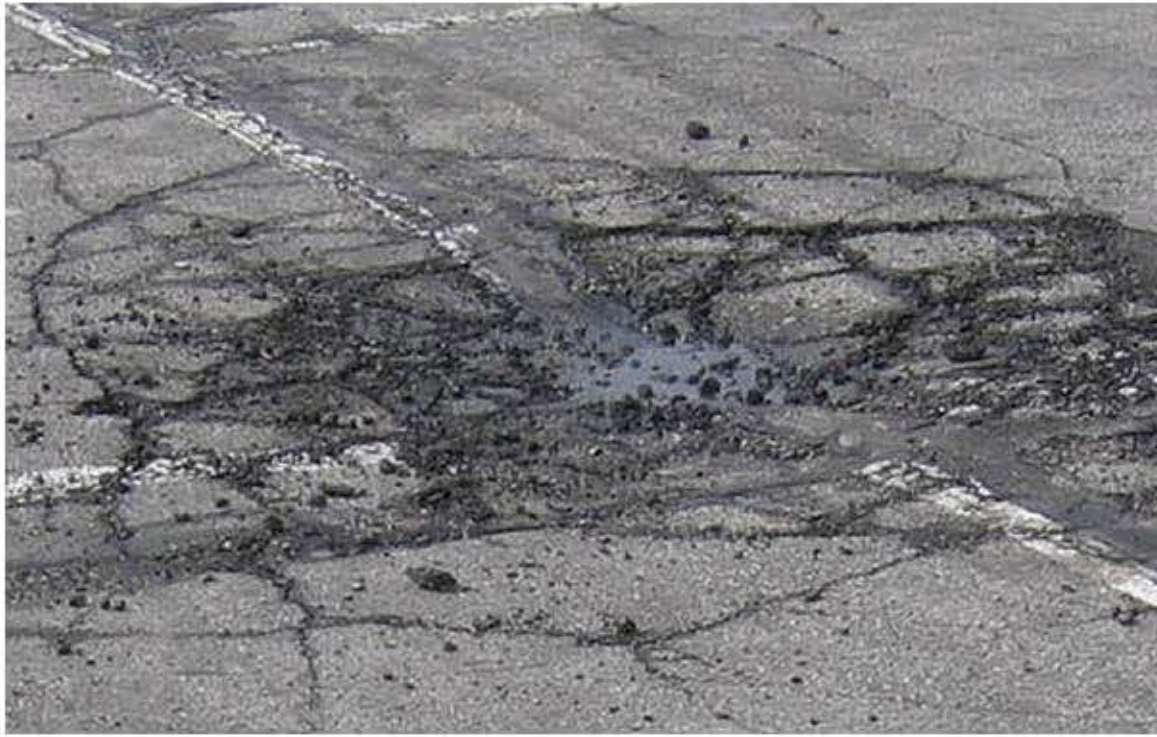
Alligator Cracking
